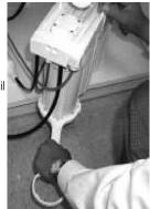
Step D – For more leverage you may leave the RO module attached to wall of cabinet. If you are unable to access the module while it is mounted, remove it prior to changing filters. Starting with the closest housing (Stage 1), remove it by turning it clockwise (left), empty water, then discard filter. Continue on to the 2nd housing (Stage 2) and 3rd housing (Stage 3).
