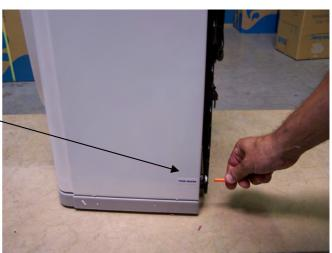
2.6 Connect supplied orange feed water tubing to feed connector on back of cooler.
