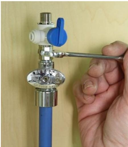
2. Now install the whip hose or tubing on the angle stop valve and tighten.
