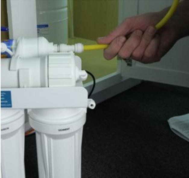
3. Connect orange tubing from the angle stop supply valve to RO unit at the sediment filter inlet fitting.
