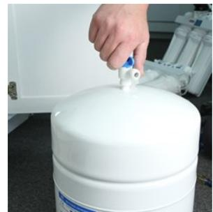
2. Install the tank valve by turning it clockwise. Tightening it hand tight is usually adequate but additional tightening may be required.
