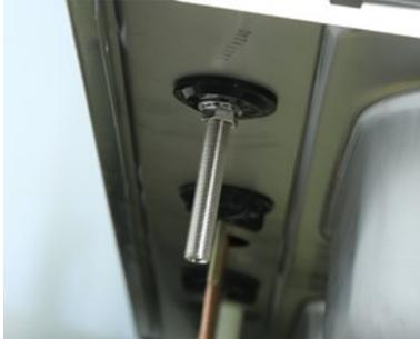
2. Once the faucet is secure, install the 7/16" UNS x 3/8" QC faucet connector on the threaded nipple. This fitting doesn't require sealant. This fitting will seal at the beveled surface. Tighten the fitting hand tight then an additional 1/2 turn with a wrench or pliers.
