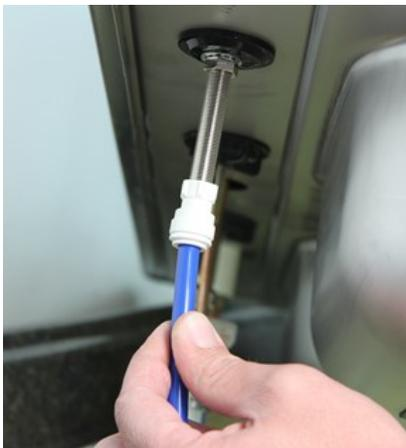
4. If an air gap faucet is being used continue to the next steps. Push the 1/4" drain line from the RO module on to the smaller brass barb on the bottom of the faucet. Be sure the tube is completely pushed on the barb or a leak could occur.
